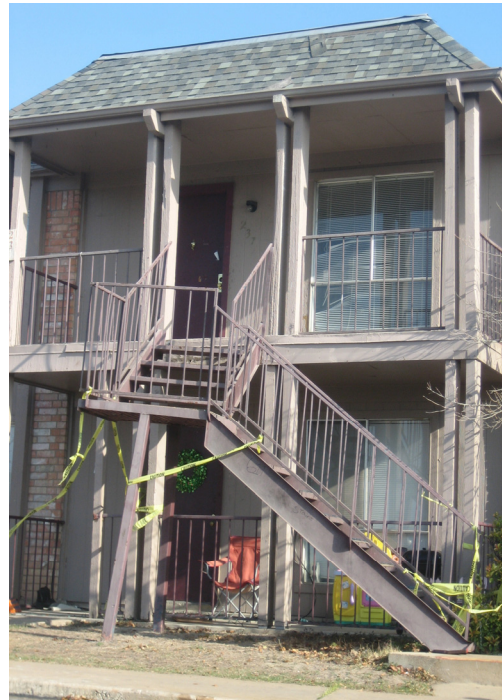
A potential code violation
